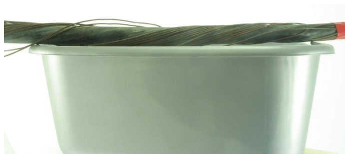
Figure 2: Place a basin under the cable to catch leaking fluids.
