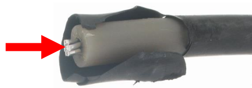
Figure 4: Insulation shield is not bonded to the insulation.
