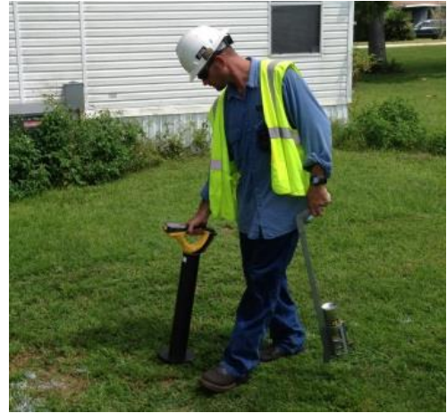
Figure 6: Use an RF locator to pin-point the location of all splices on the circuit.
