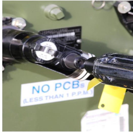
Figure 13: Install the permanent cap at the receiving end of the cable.
