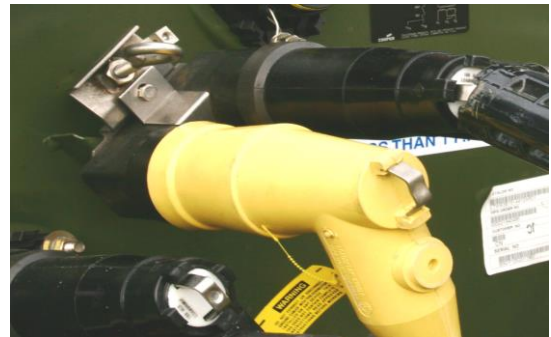
Figure 2: Ground the cable and make safe to work.
