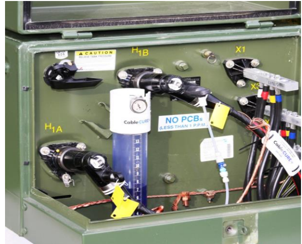
Figure 14: Re-install the feed tank for the 60-120 days soak period.
