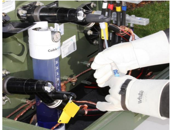
Figure 11: Connect the feed tank to the cable by connecting the QDs and secure within the enclosure.
