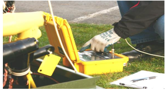
Figure 4: Perform TDR test to identify splices and neutral corrosion and to measure the cable's length.
