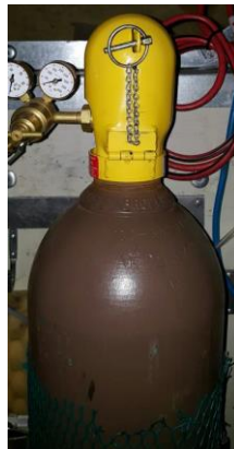
Figure 11: Cylinder with protective safety cap installed.
