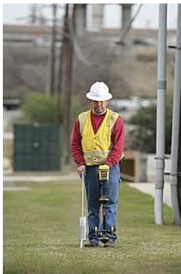
Figure 5: Walking the cable length.
