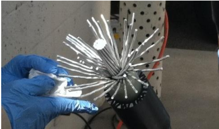
Figure 28: Cleaning the strands with solvent and rag for light corrosion.
