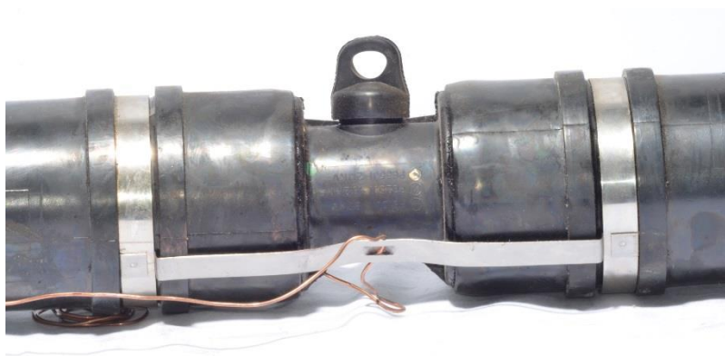
Figure 70: The brace installed.
