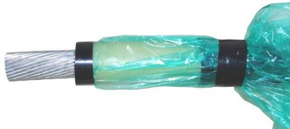
Figure 31: The insulation is protected from debris created from the cleaning process.
