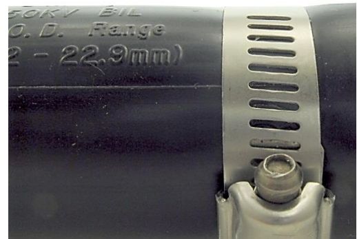
Figure 8: Clamp body even with splice body.
