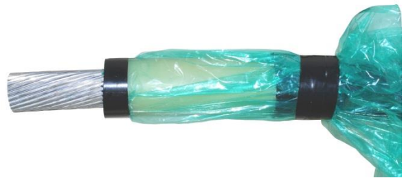
Figure 17: Protect insulation from debris.
