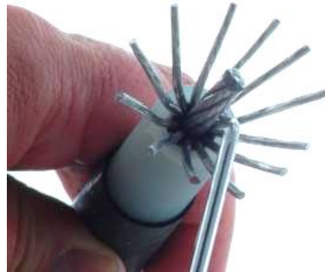
Figure 15: Fan the outer strands and remove grease or oxides.
