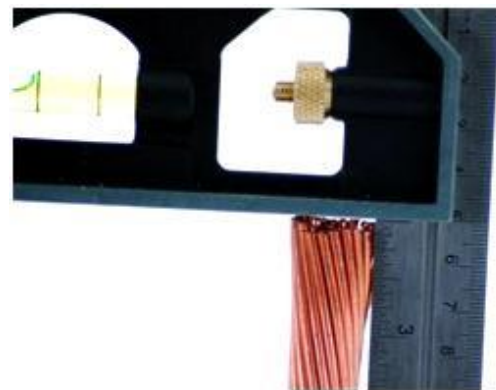
Figure 11: Square the conductor strands.
