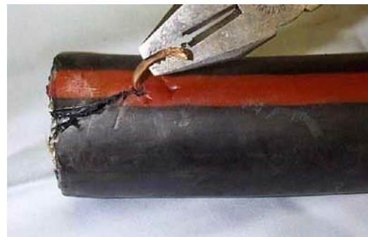
Figure 2: Use pliers to start the concentric neutrals.
